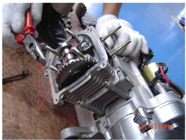
Fig. 10. Install alignment pins
